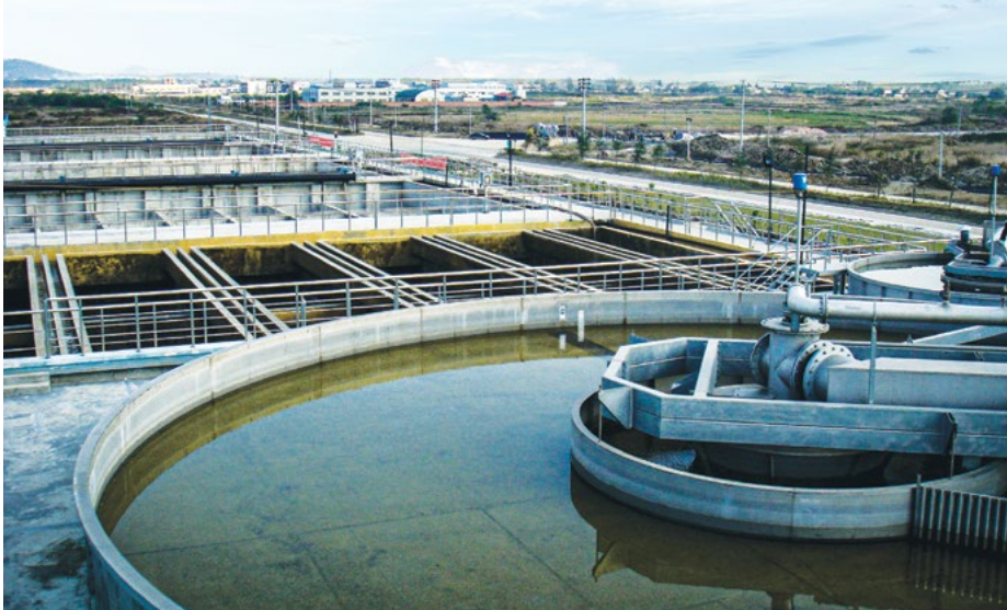
One of the wastewater and reclaimed water treatment plant facilities at the Amata Industrial Estate in Thailand
