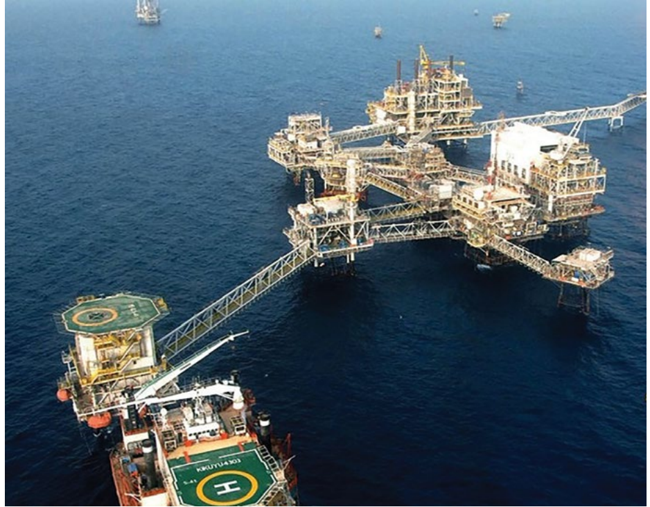
RW project of ISND, China
