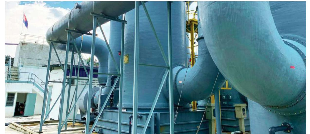
Air stripper and gas scrubber with treatment capacity up to 500 ppm of ammoniacal nitrogen content operation at Pollutant Removal System ("PRS") Simfang Renggam Water Treatment Plant
