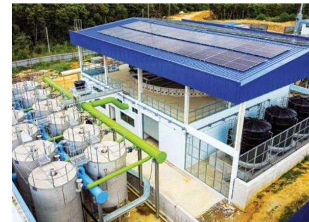
63 kWp solar panel installation at Sultan Iskandar Water Treatment Plant extension project
