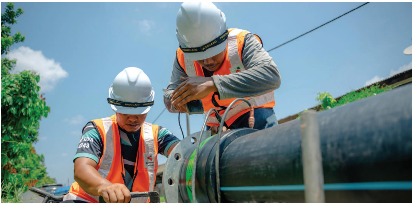
RTSB employees conducting quality inspection on HDPE pipe jointing to ensure reliable water supply to customers
